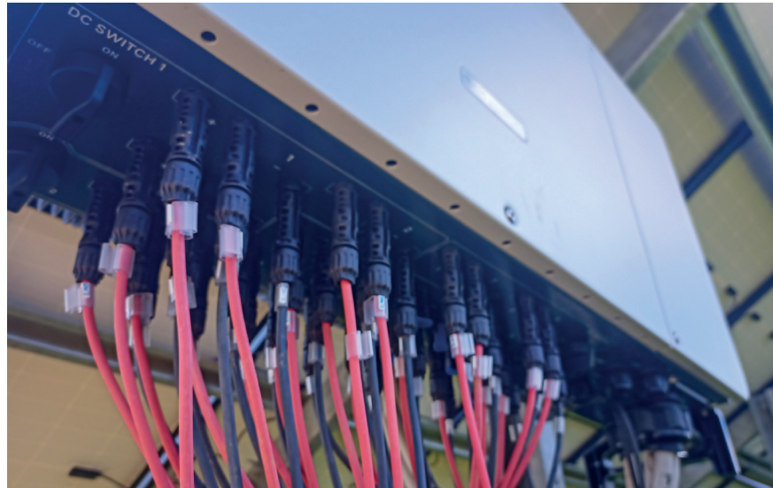
SG250HX inverters have 12 MPPTs for a total of 24 string inputs.
